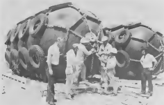
Prior to positioning the rubber fenders to the Medium Size Tanker, the fenders have to be inspected and wires attached to them. Above, from left to right, B. van Duin, P. Loeftop, E. Dubero, A. Ponson, E. Ridderstap and J. van der Linde.
